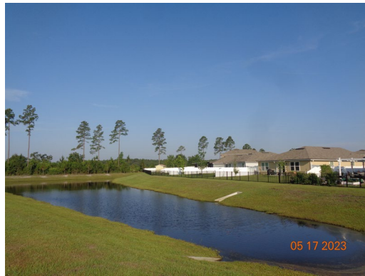
Pond 8: No algae noticed, pond level is low. There is evidence of the grass carp pulling up the spike rush throughout the pond.
